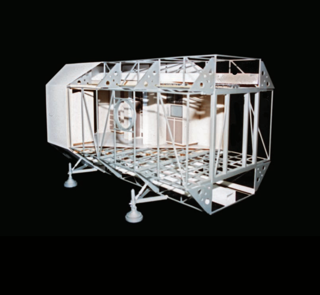
CONSTRUCTION CONCEPT FOR ANTARCTIC FACILITY MODULE
