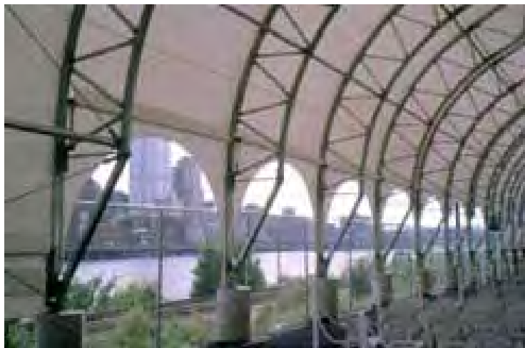
Construction Uses “Off-the-Shelf” Trusses
