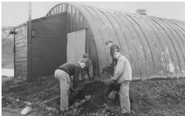
Weather Proofing a Nissen Hut
