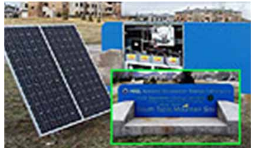
These two silicon modules are rated at 50 watts each, and generate power to illuminate a large entry sign.
