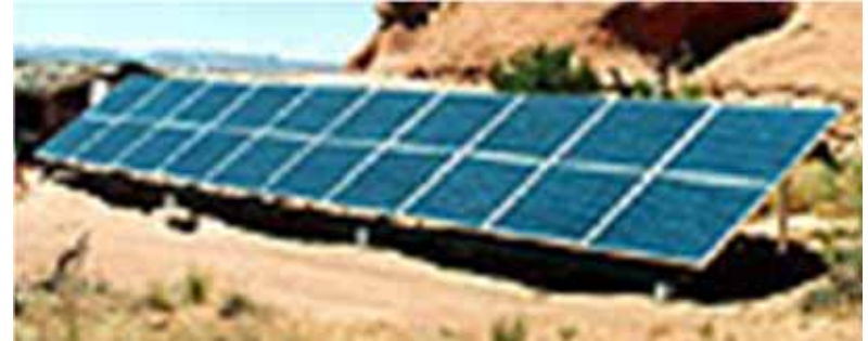
This 6.5 kilowatt PV array supports an all-purpose general store, restaurant, gas station and public campground near Moab, Utah.
