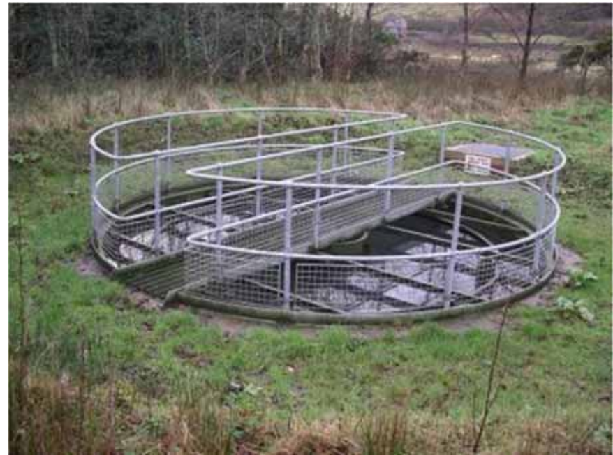
Primary Sedimentation Tank at a Rural Sewage Treatment Plant
