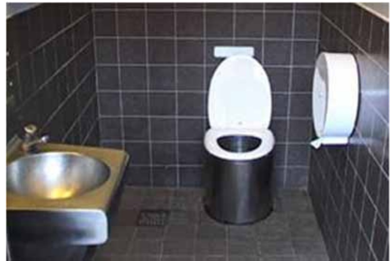
Public Compost Toilet Installation Along a Highway in Sweden.
