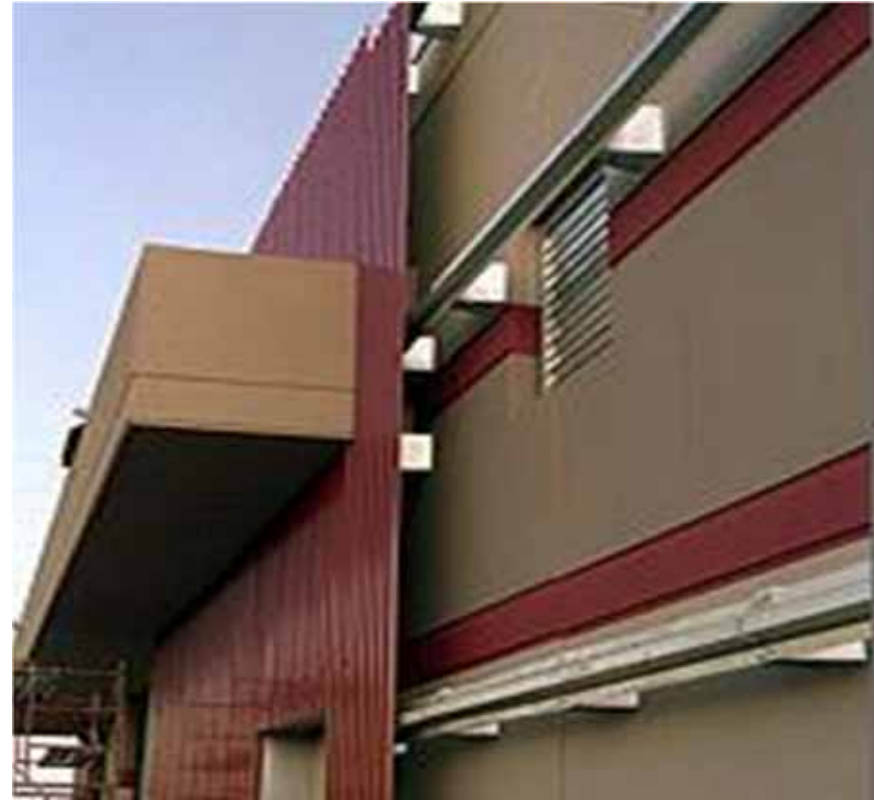
Transpired Collector at the Denver FedEx Building for Space Heating
