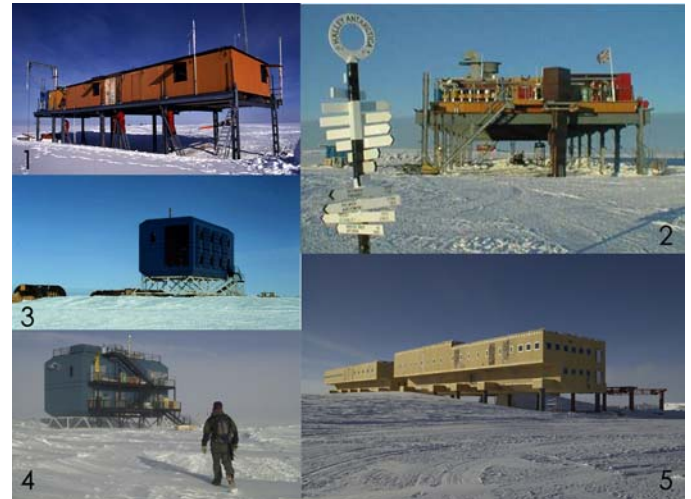
Figure 2: Antarctic Elevated Stations. (1-Filchner station, 2-Halley station, 3,4-Atmospheric Research Observatory, 5-Amundsen-Scott Station)
